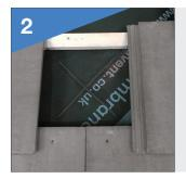
Remove the tile where it is to be replaced with an Ulti-Line Tile Vent and Mark the cut line as shown
