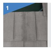
Set out the roof and lay the tiles in line with the manufacturers fixing instructions until you reach the area where the vent tile is to be fitted
