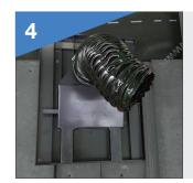
Select the Vent Tile to match to profile and colour and fit either without a flexipipe (if just being used for roof ventilation) or with a Ulti-Mate Flexipipe ULTI3FP for connection to Soil Pipe of Mechanical Extraction
