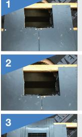
Decide position where vent is to be installed, cut and mark membrane and cut Slates 125mm width and 230mm from top
